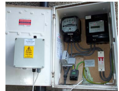
M62 mounted in a meter cabinet
